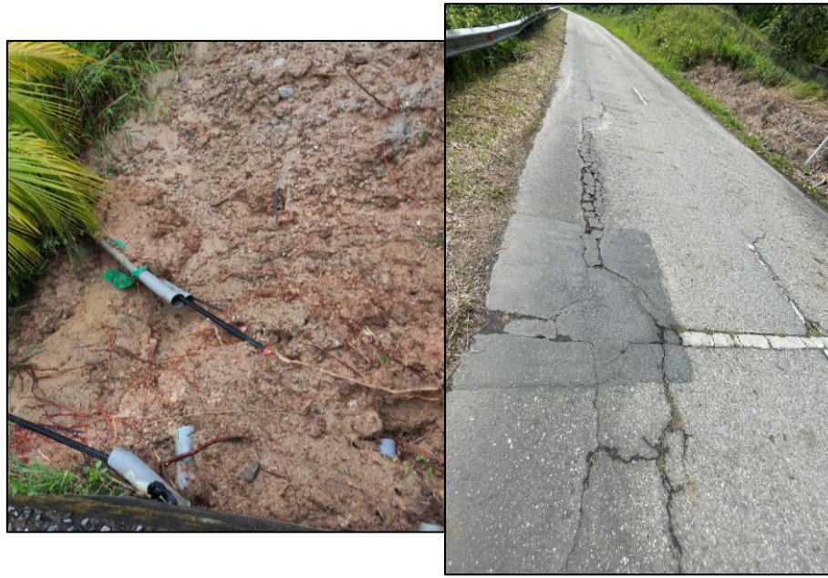
Figure 7 Evidence of underground soil movement in AOI 1.
